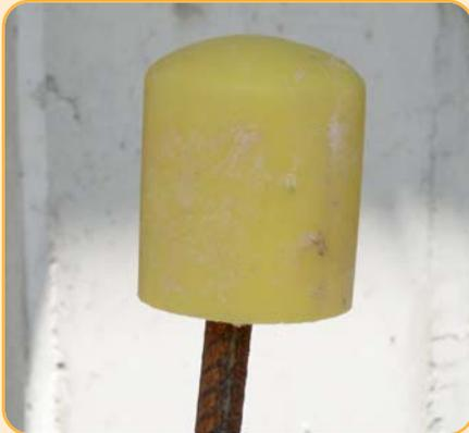
Recent research conducted by the NSW Plant Consultative Committee has shown that plastic caps fitted to the ends of exposed steel reinforcement bars may offer little protection against serious workplace accidents, including impalement.
