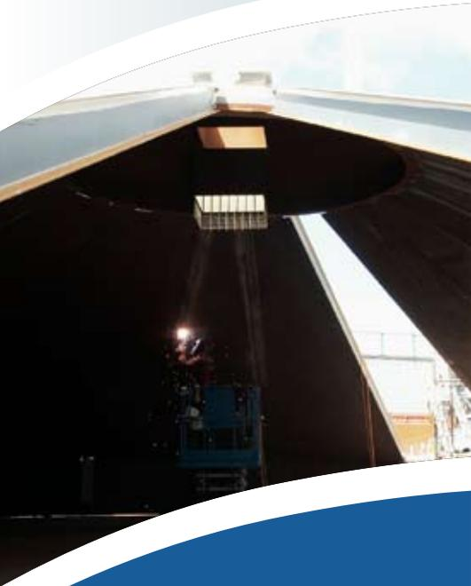
The majority of the shell and cone sections of the storage cells have been fabricated from 250 Grade XLERPLATE® steel. Ring beam sections and columns have been fabricated from 350 Grade XLERPLATE® steel.
