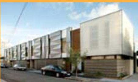
Unlike the vast majority of COLORBOND® steel applications in residential architecture, the cladding on these townhouses is folded, and resembles origami on a grand scale. Five of the six townhouses are clad with these folded steel sheets, while the sixth is clad with corrugated fibreglass, emulating typical industrial roofing.
