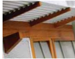
The Nobbs Blyfield development in Maylands, South Australia added a contemporary and environmentally-friendly backyard extension to a 1900s inner suburban villa. Troppo Architects chose framing, roofing and wall cladding made from BlueScope Steel's ZINCALUME® steel for the home extensions.
