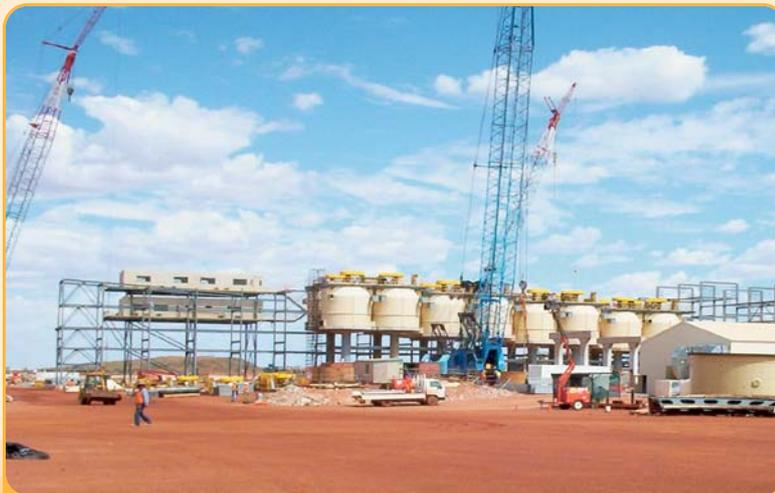
*JV Engineering's flotation tanks at Telfer Mine.*
