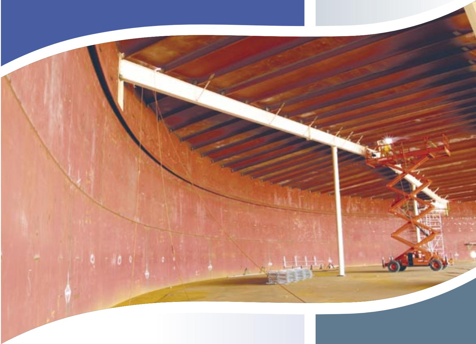
Internal surfaces of the tanks are coated with a special "high-build" epoxy layer developed for contact with drinking water.
