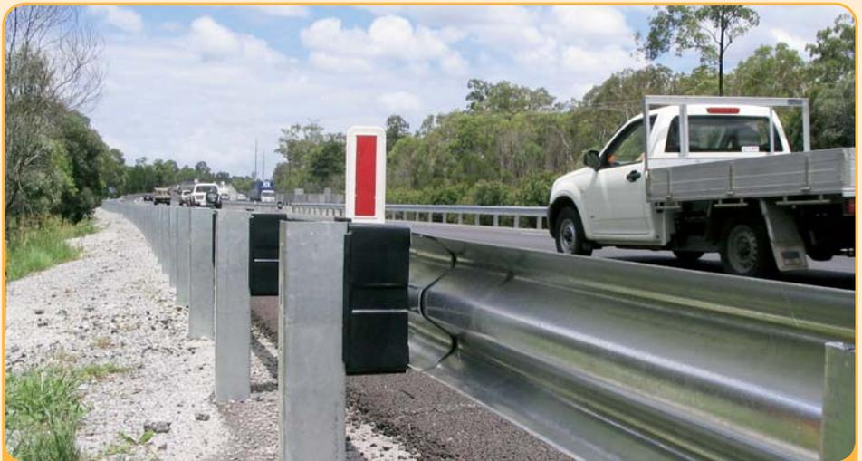
*FX-350 is an advanced W-beam safety barrier.*
