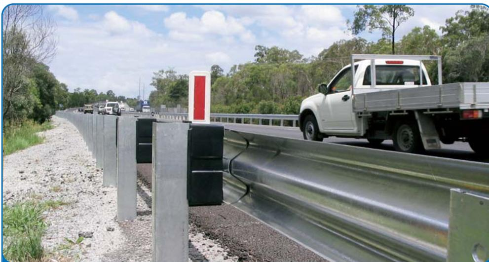
FX-350 is an advanced W-beam safety barrier.
