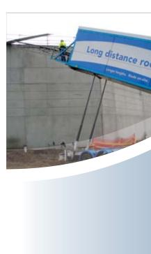
A unique sled arrangement allowed the tails of the 47.3 metre ridge-to-step sheets to be linked to the heads of the step-to-gutter sheets, simplifying the installatiion process.
