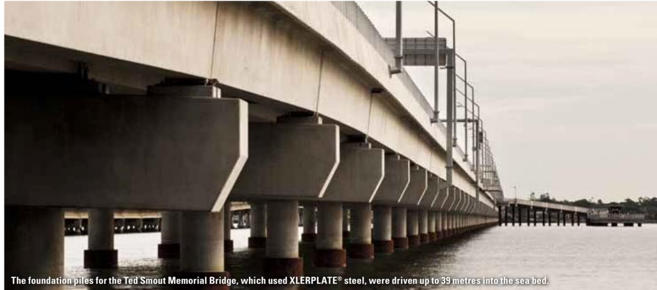
The foundation piles for the Ted Smout Memorial Bridge, which used XLERPLATE® steel, were driven up to 39 metres into the sea bed.
