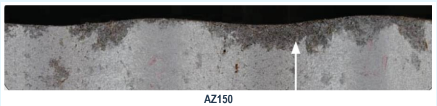
Figure 2: Unpainted sheltered walling (i.e. unwashed) in a severe marine environment after 50 months.
