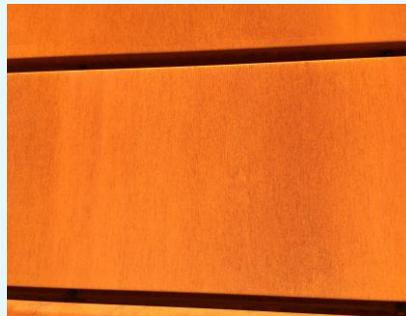
In situations where one surface of a REDCOR® weathering steel structure receives more exposure than the other there is likely to be a difference in appearance between the two surfaces. The more boldly exposed surface will form the patina more rapidly, whereas the protected surface will form the patina more slowly and have a rougher surface texture than the exposed side.
