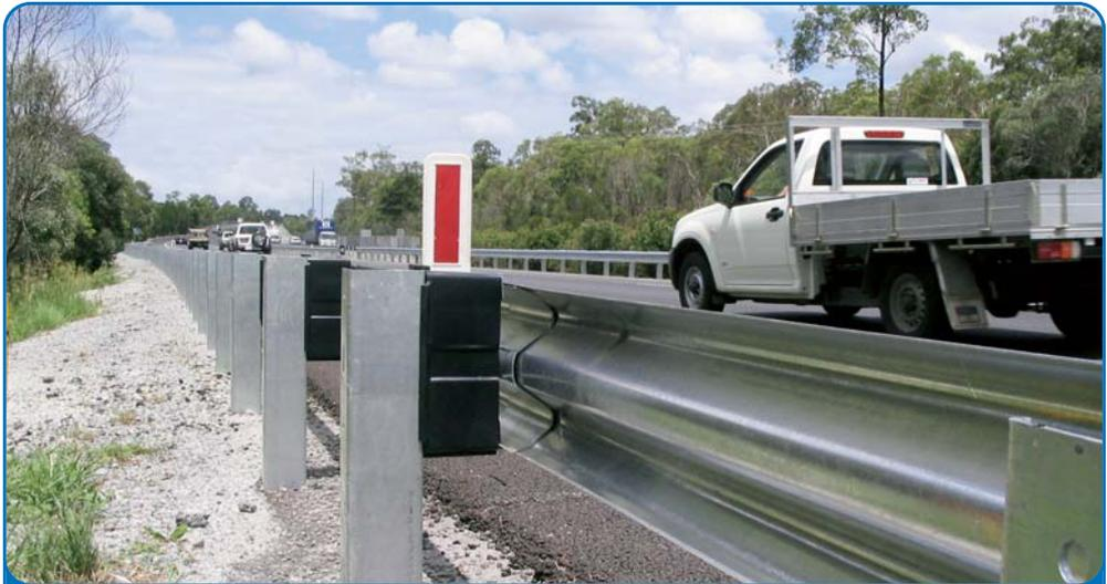
*FX-350 is an advanced W-beam safety barrier.*
