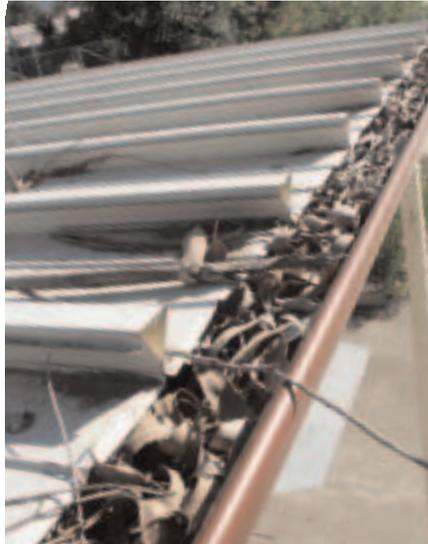
1) A typical suburban gutter clogged with leaf litter prior to cleaning.
