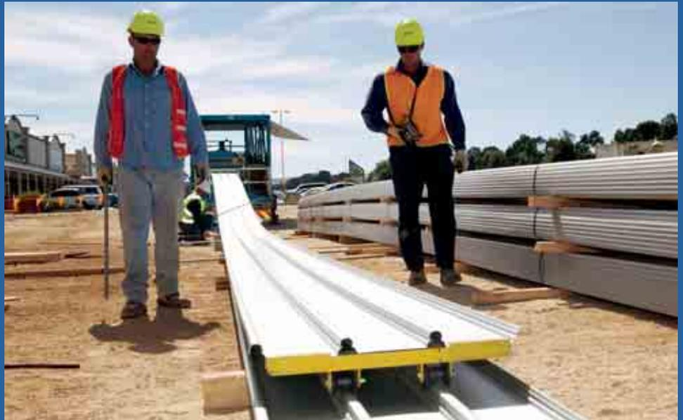
BlueScope Lysaght's mobile rollforming capability offers numerous unique benefits to its customers, Bill says. "Our flexible operating capacity – the mobile rollformer has a tilt capability – allowed material to be delivered directly onto the roof, creating savings in craning and labour costs," he says.
