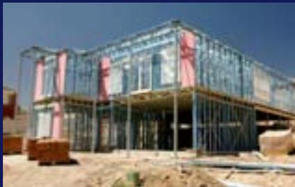
Building frames made from TRUECORE® steel are quick and easy for builders to put up, and are ideal for open space contemporary designs because of the product's excellent spanning capabilities.
