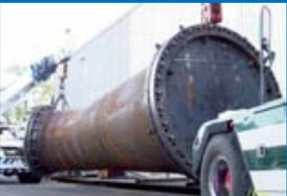
"Some of the pipes are 6 metres long with a diameter of 2.7 metres so they're three times as big as a car," he said. "We delivered 28 truckloads to Warragamba Dam, and most were over-dimensional – some single loads weighing close to 20 tonnes."
