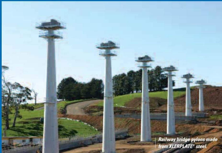
*Railway bridge pylons made from XLERPLATE® steel.*
