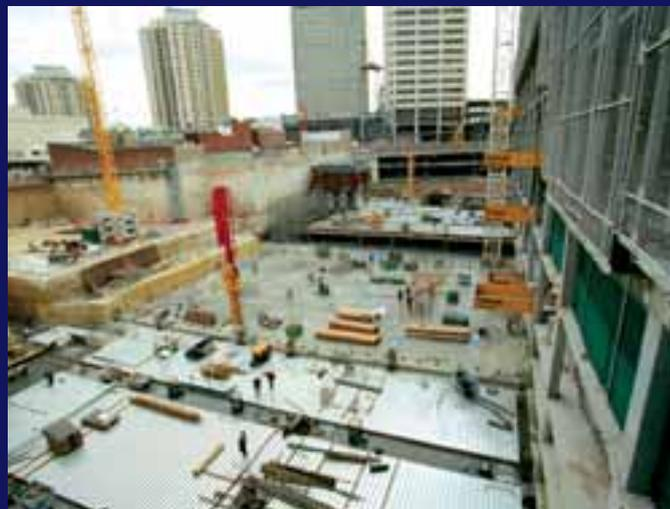
Formwork contractors Dolso & Wideform are installing the permanent steel formwork as slab formwork while using conventional formwork for the band beams. Sydney post-tensioning specialist Austress Freyssinet Pty Ltd are responsible for the post-tensioned system used at Westfield Bondi Junction.
