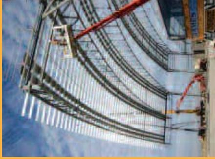
The system uses conventional trusses manufactured from square and rectangular hollow sections which are stressed with high tensile cables to provide added strength.
