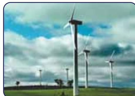
**Wind towers made from XLERPLATE® steel.**
