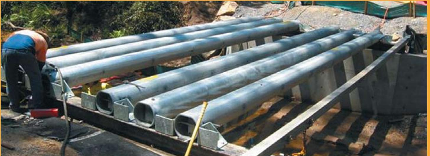
*Flat sections on opposite sides of TRANSISPAN® girders spread loads and simplify installation.*
