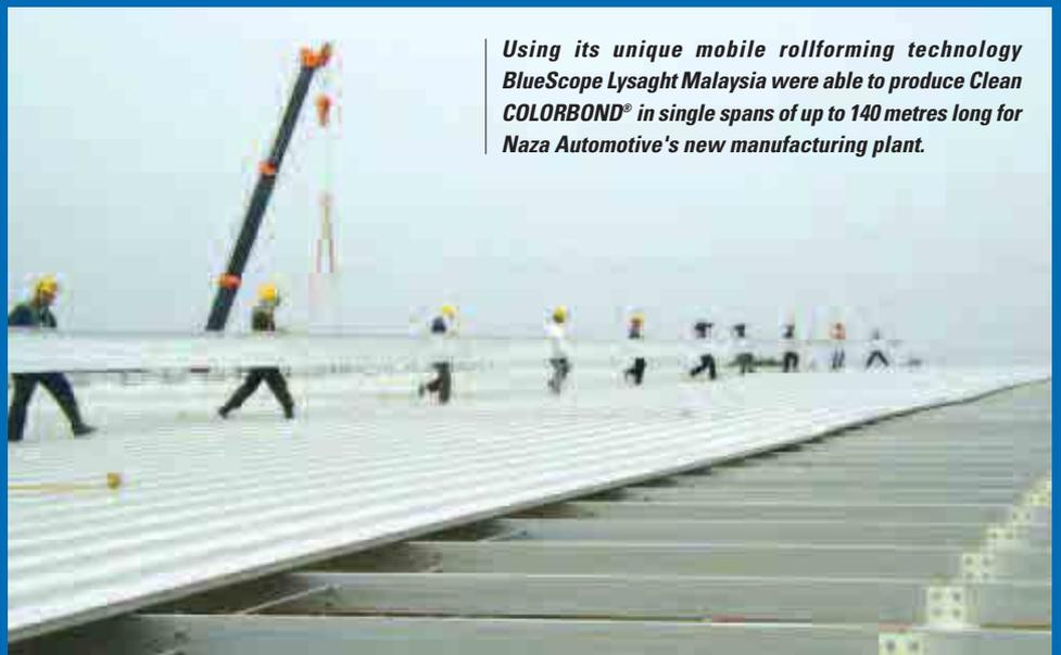
*Using its unique mobile rollforming technology BlueScope Lysaght Malaysia were able to produce Clean COLORBOND® in single spans of up to 140 metres long for Naza Automotive's new manufacturing plant.*
